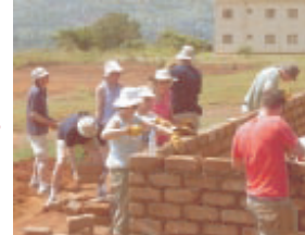
Building a wall in Uganda
